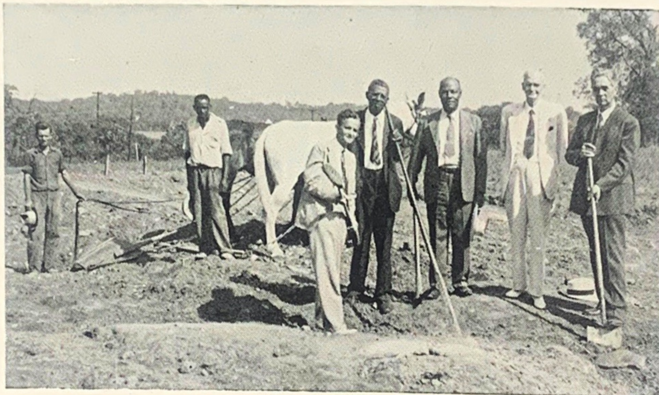
GROUND BREAKING OF THE J. B. LAWRENCE BUILDING
